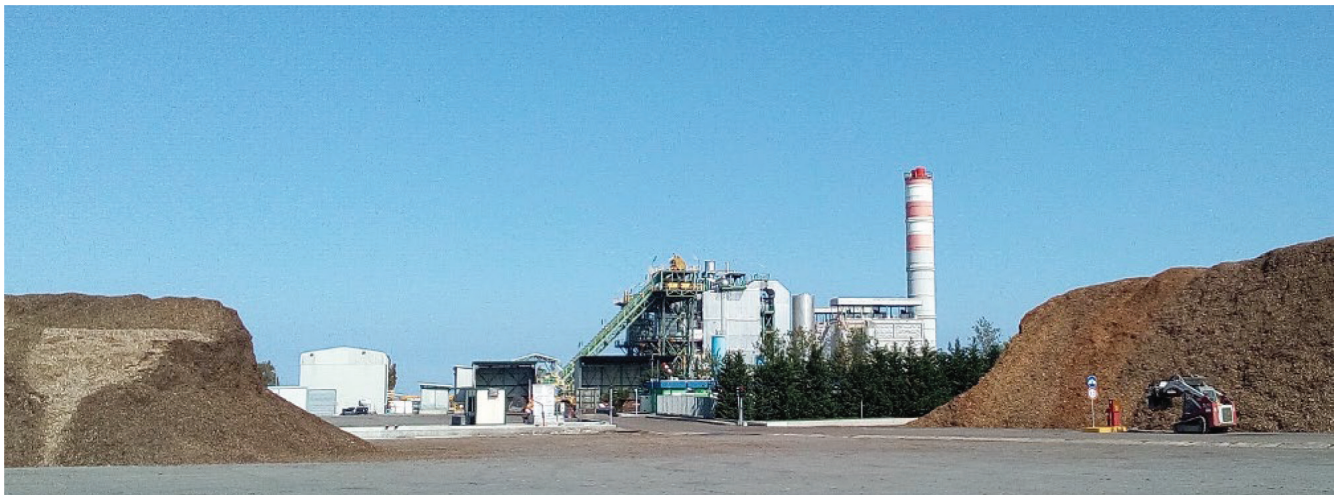
Figure 1 Biomass power plant and wood chips stored at the wood park
